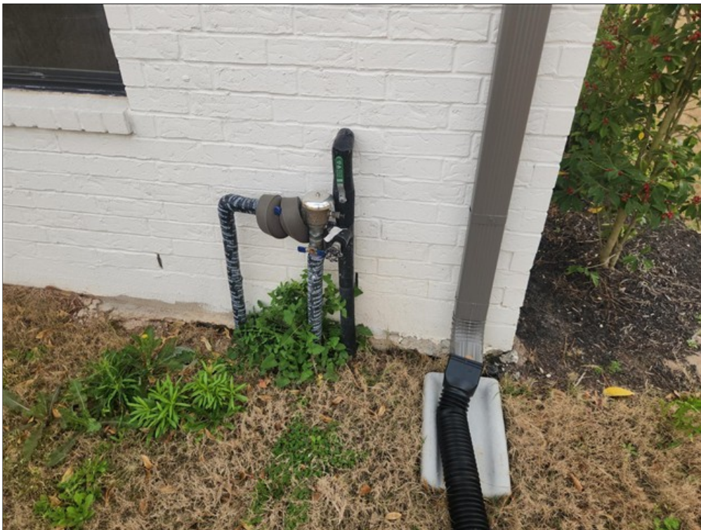
A. System vacuum breaker
