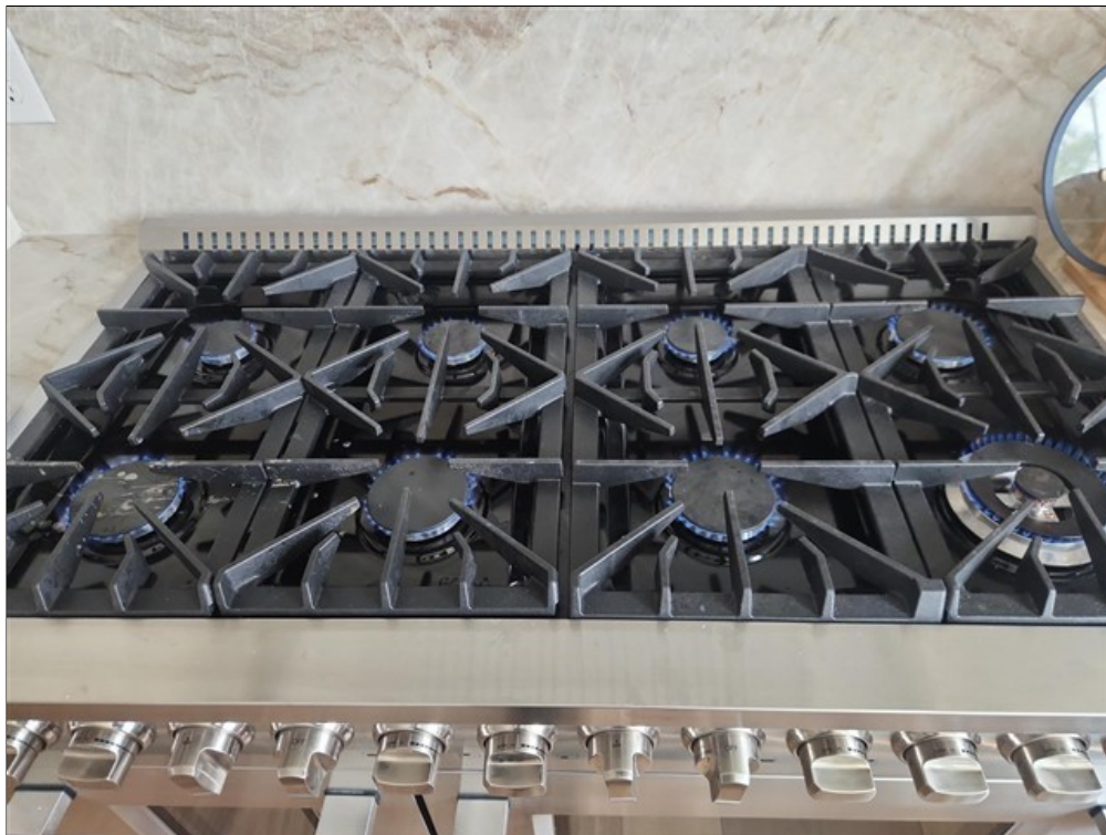
D. Burners serving cooktop have low flame when on highest gas setting
