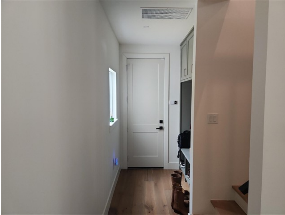
G. Occupant garage door not equipped with self closing hinges
