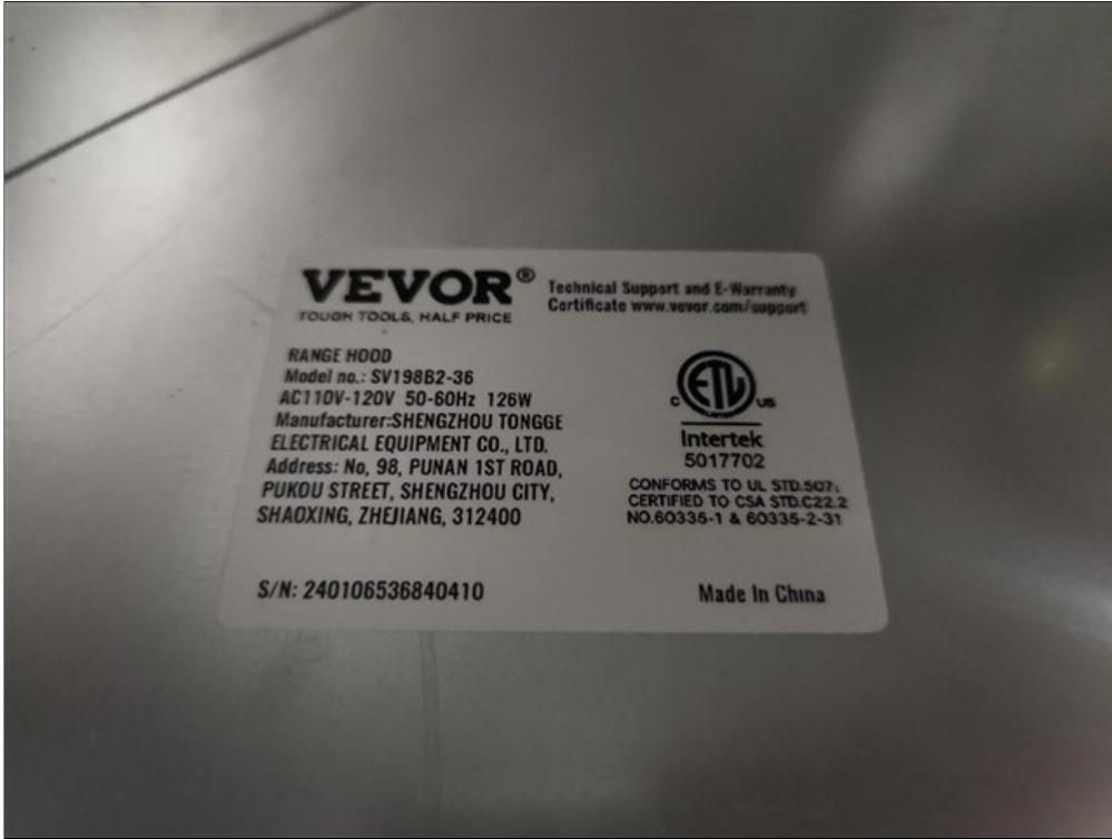
C. Range hood vent data plate
