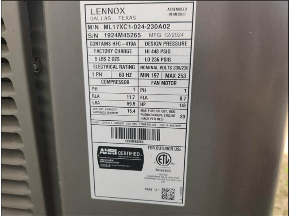
B. Condensing unit data plate
