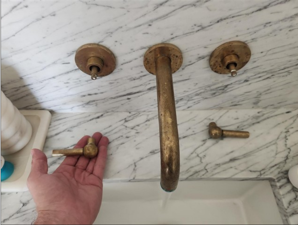
A. Detached sink water valves
