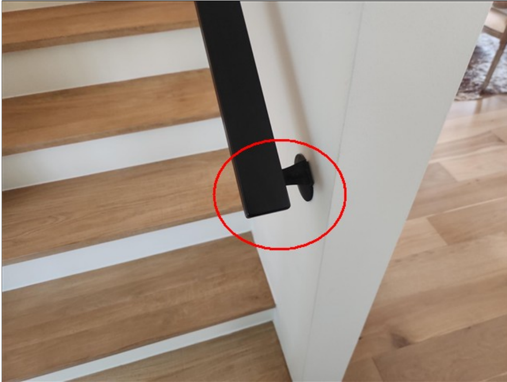
I. Hand rail does not terminate to wall or newel post
