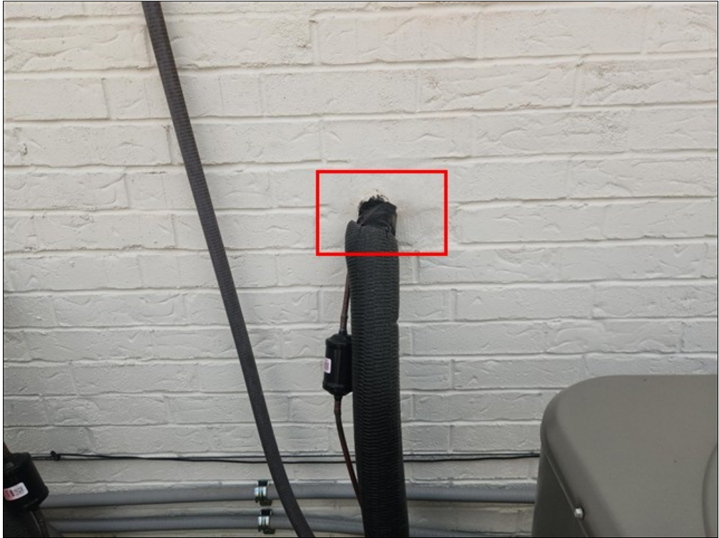
B. Refrigerant hood needed
