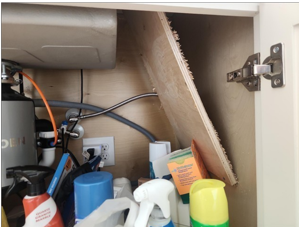
A. Unusually large "braces" installed in kitchen cabinet to support sink
