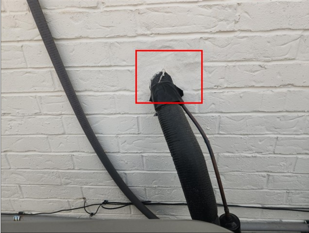
B. Refrigerant hood needed
