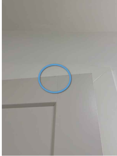
2nd Floor Guest bathroom
