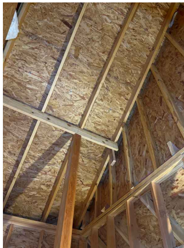
Roof structure stick built
