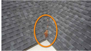
Roof surface, multiple areas
