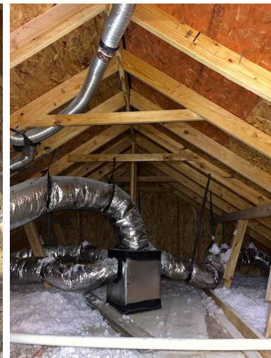
Roof structure stick built
