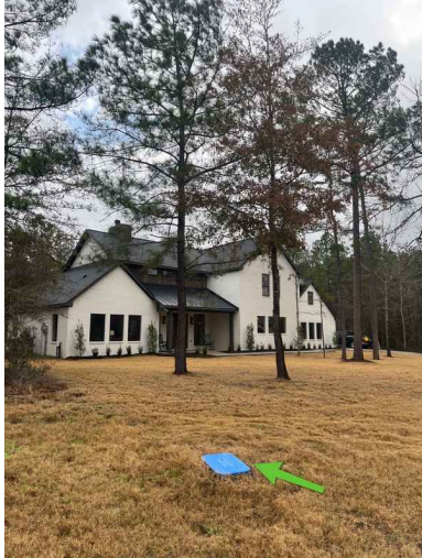
Water meter, located front left side of home
