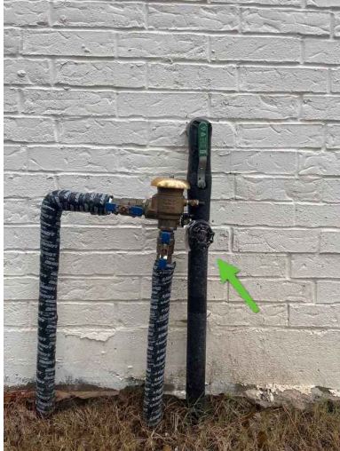
Water main shutoff, located left side of home
