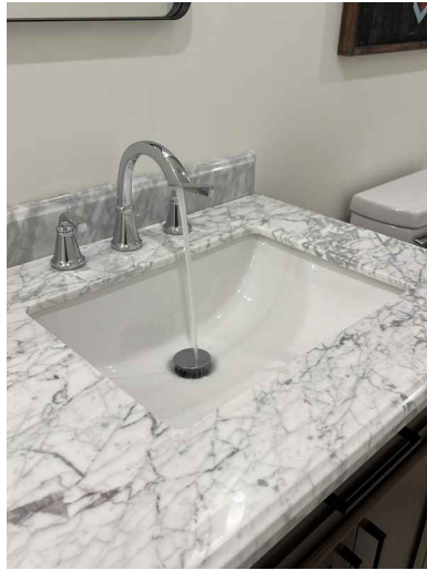
2nd Floor Guest bathroom
