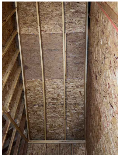
Roof structure stick built
