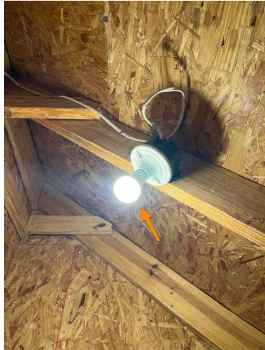
Walk in attic
