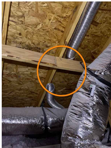
Second floor attic
