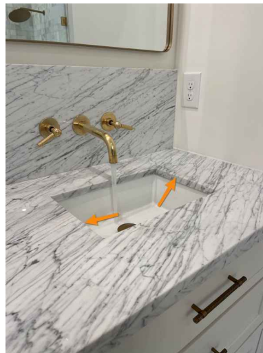
Master bathroom, right sink
