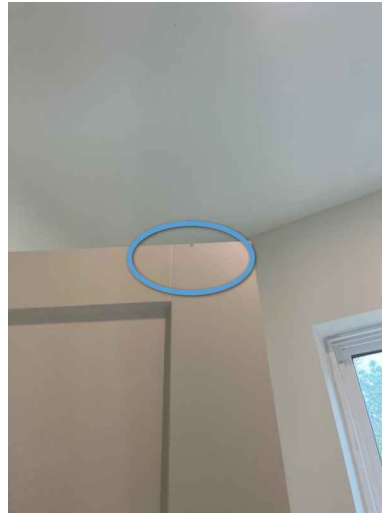
Guest bedroom closet, rear of home
