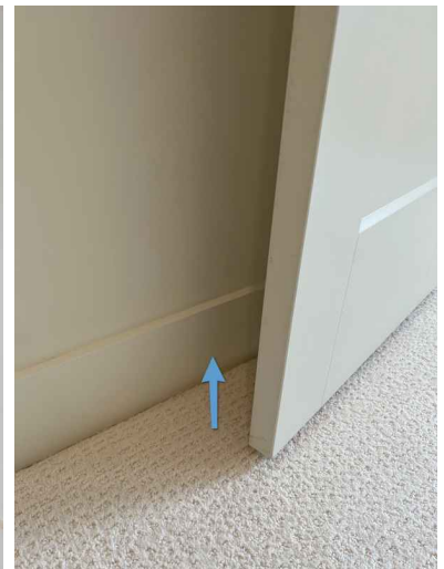
Guest bedroom closet, rear of home
